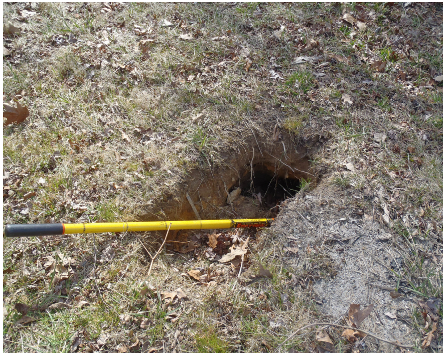
6. SINKHOLE IN SHOULDER @ SOUTHWEST CORNER
