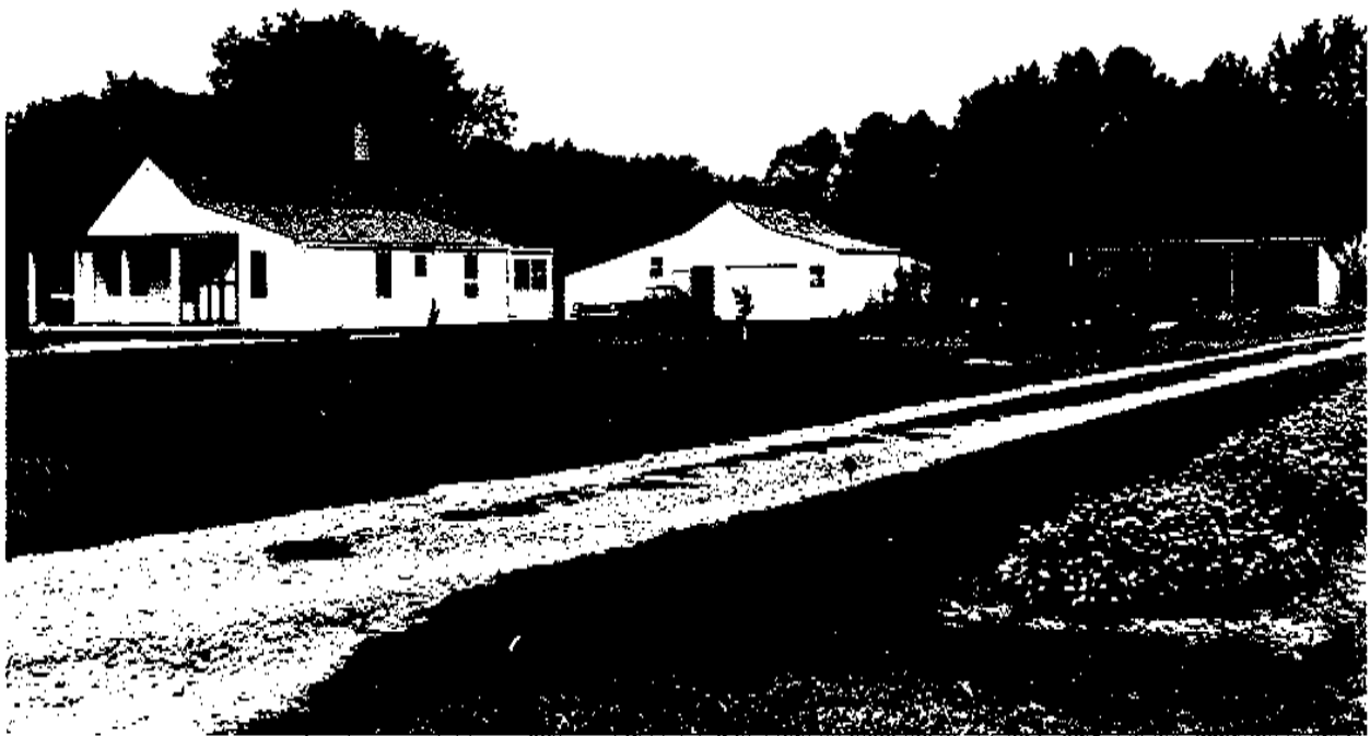
PLATE 61: Building 50, Clarence E. Wilson House, View to Southwest
