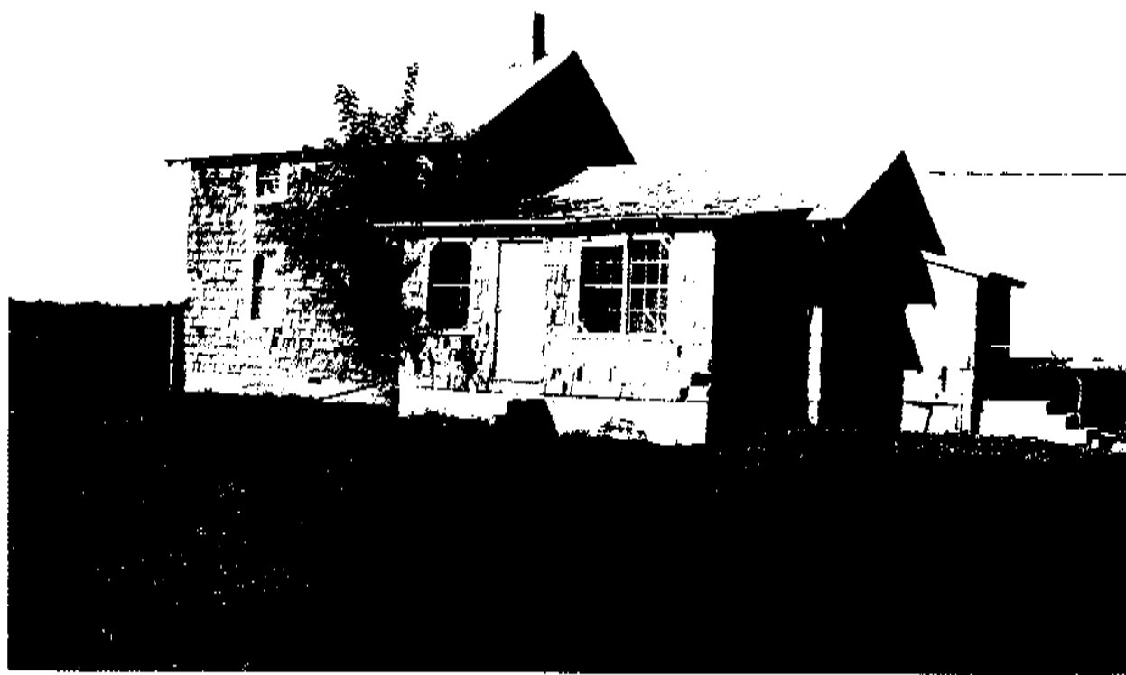
PLATE 67: Building 56, Coleman Farmstead, House, View to Northeast
