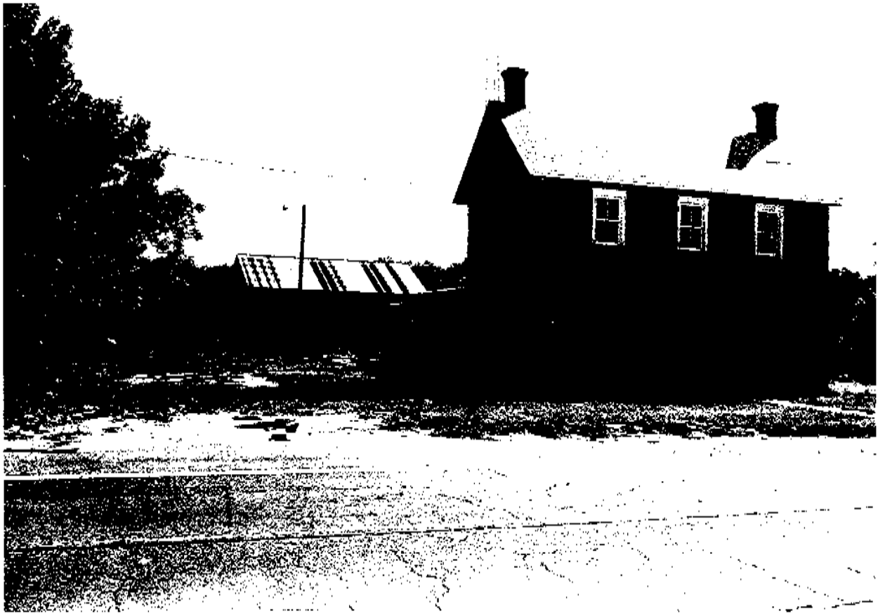
PLATE 66: Building 55, Robert Short Property, View to South
