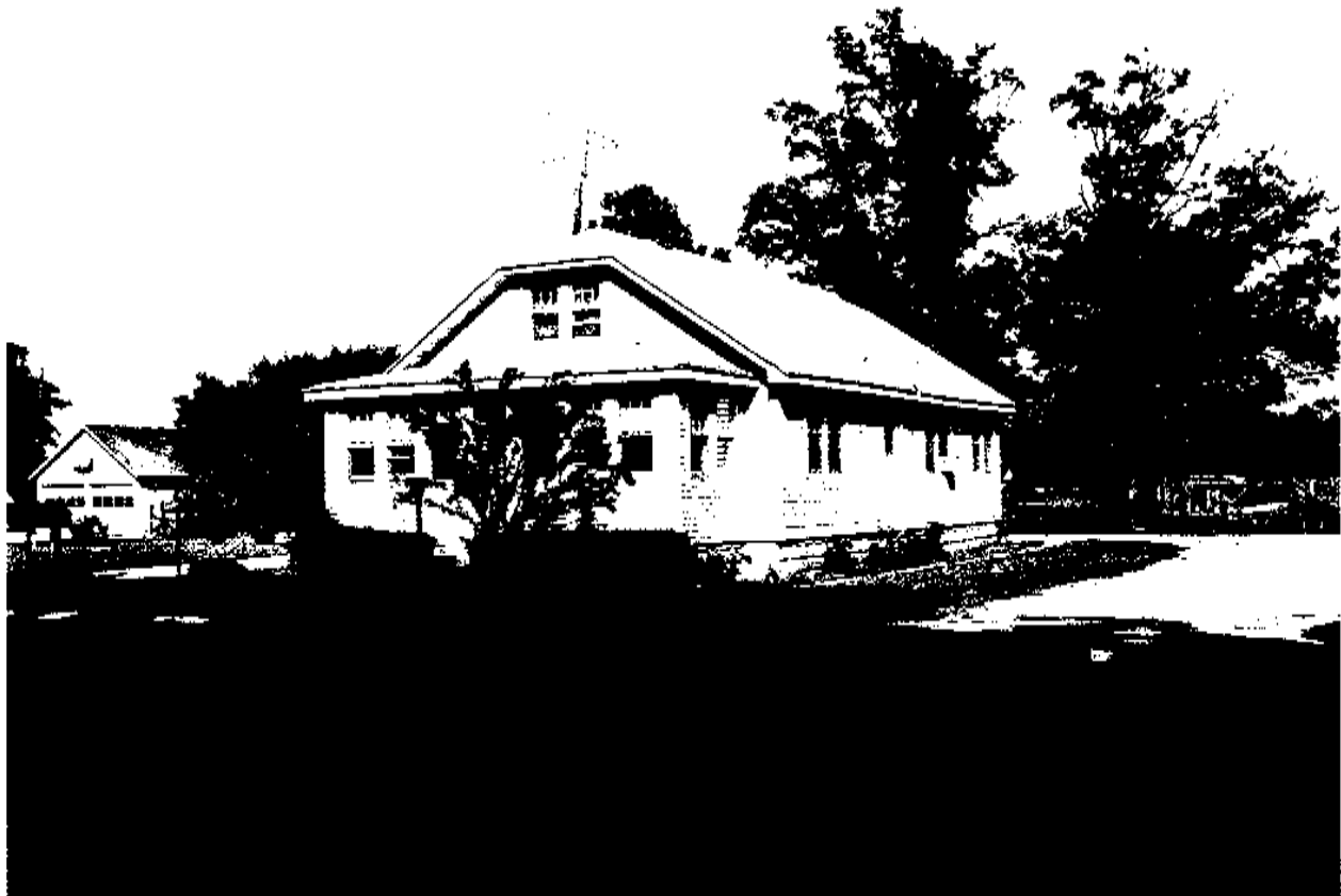
PLATE 34: Building 26, Gwendolyn Layton House, View to Northeast
