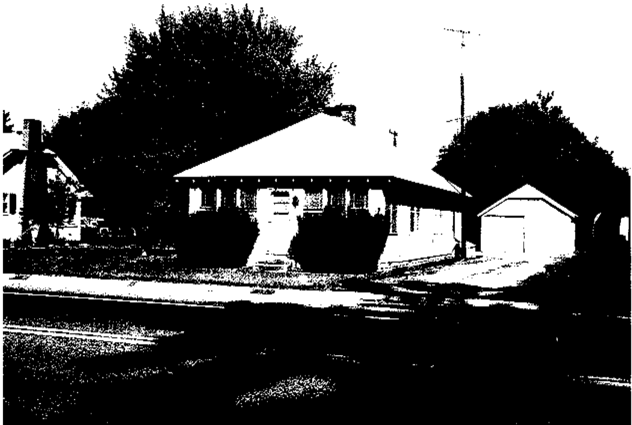
PLATE 37: Building 29, Robert Gray House, View to Northeast
