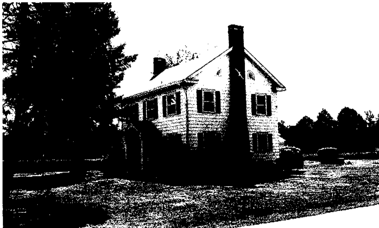
PLATE 26: Building 19, Clyde Clark House, View to Southwest
