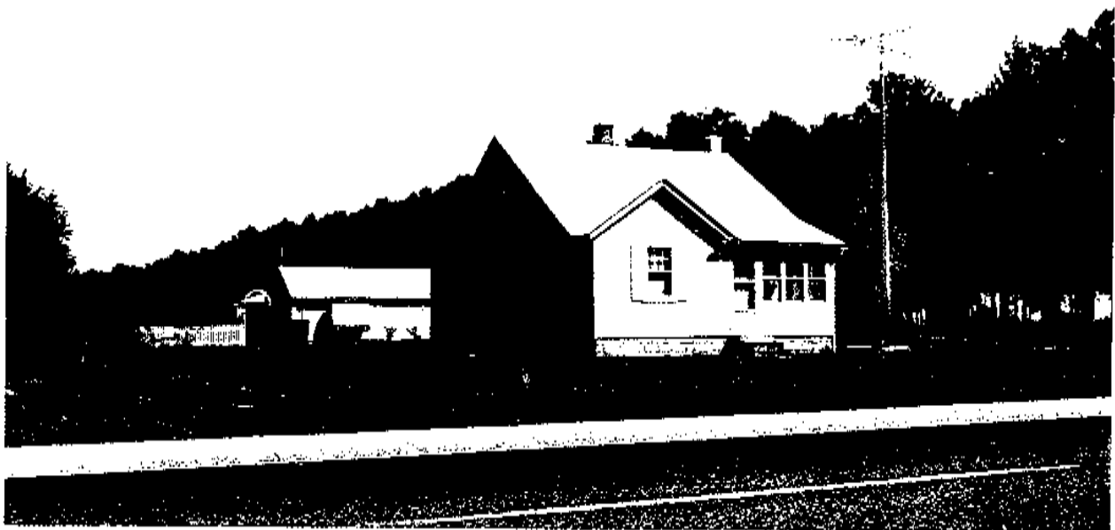
PLATE 31: Building 23, Theodore Walius House, View to Southeast (1988)
