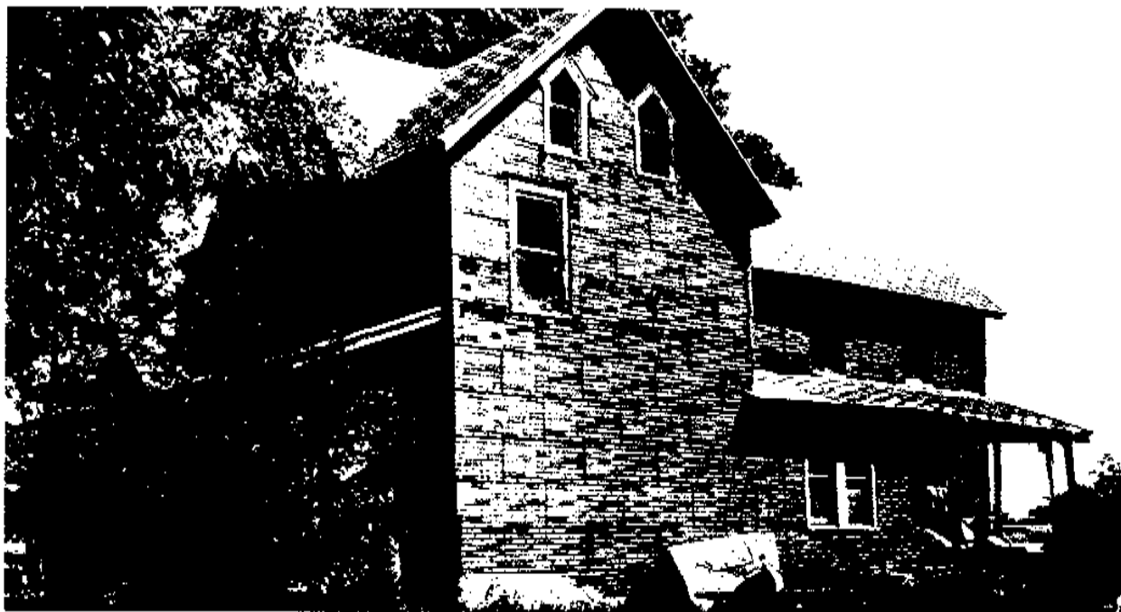
PLATE 14: Building 11, A. Carey House, View to Southeast (1988)
