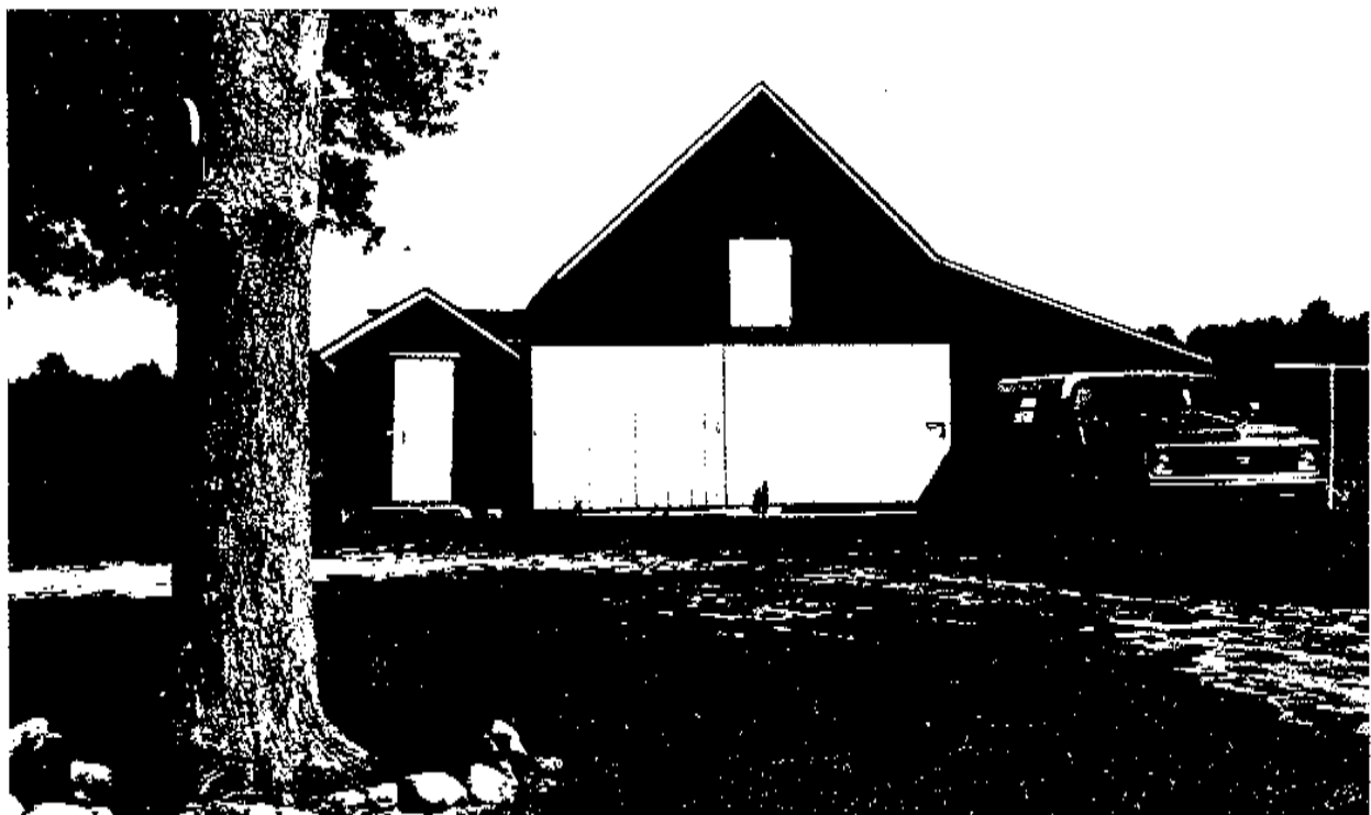
PLATE 30: Building 22, Preston Evans House, Barn/Shed Group, View to East
