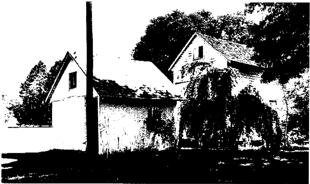
PLATE 21: Building 16, Delmarva Nurseries, Sheds, View to East (Non-Extant)
