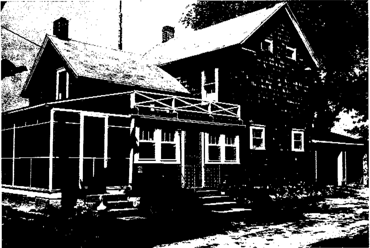
PLATE 29: Building 22, Preston Evans House, View to Northeast
