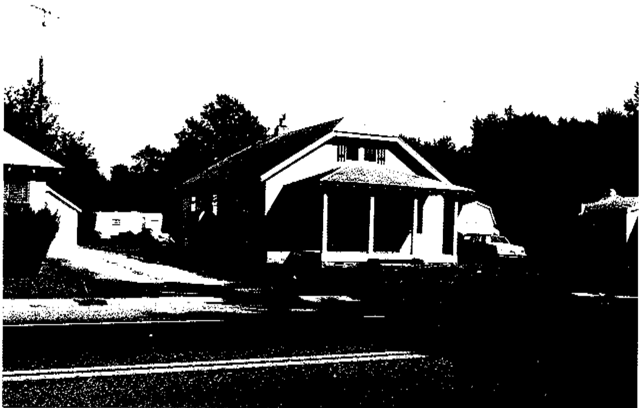
PLATE 38: Building 30, Alvin Niebert House, View to Southeast
