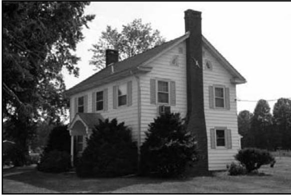
main building (.001), façade and north side view to SW
