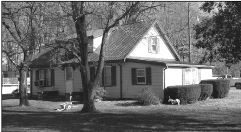
main building (.001), façade and south side, view to NE
