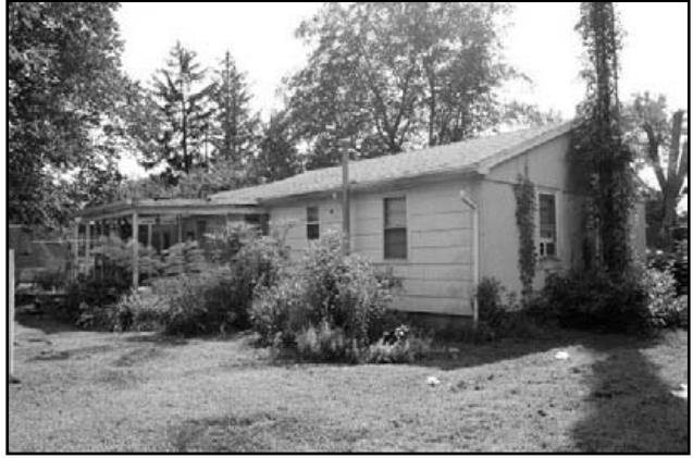
main building (.001) facade, view to SW
