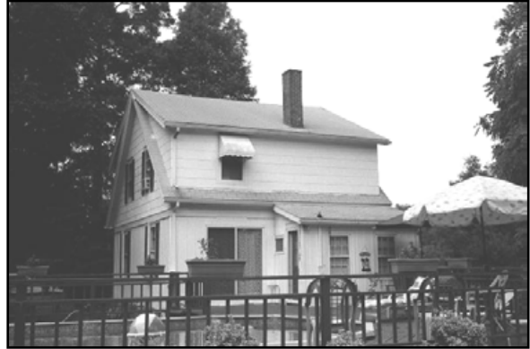
main building (.001), rear and south side, view to NW
