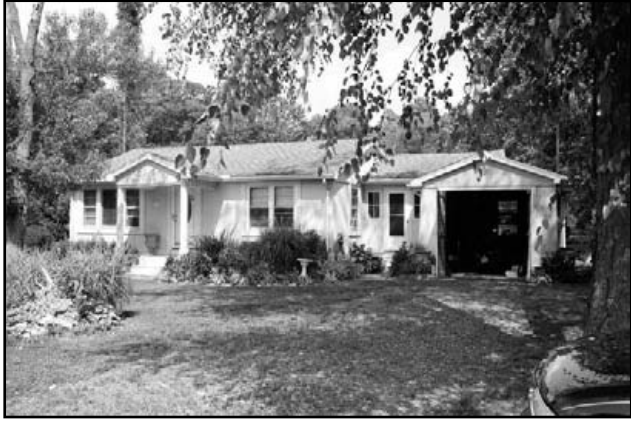
main building (.001) facade, view to E
