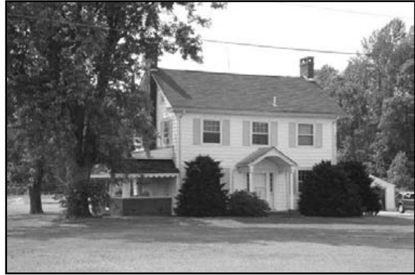
main building (.001), façade, view to W
