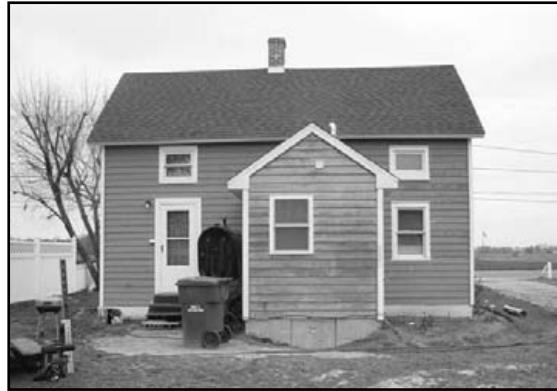
main building (.001) rear, view to N
