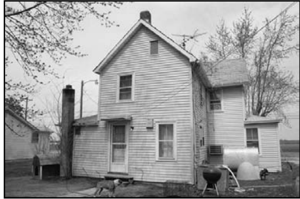
main building (.001) rear, view to NW
