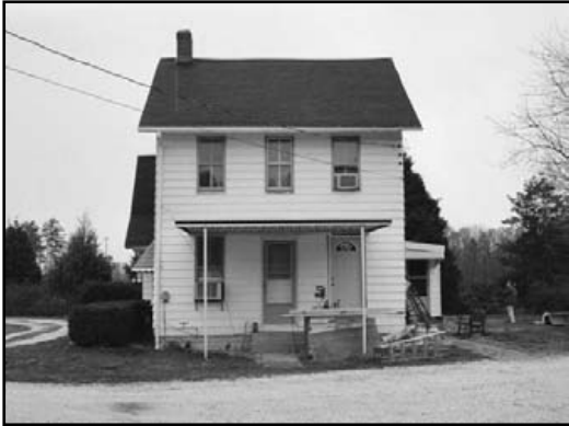
main building (.001) facade, view to N
