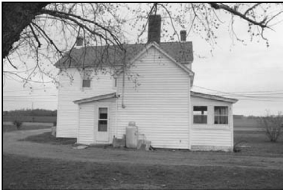
main building (.001) rear, view to N
