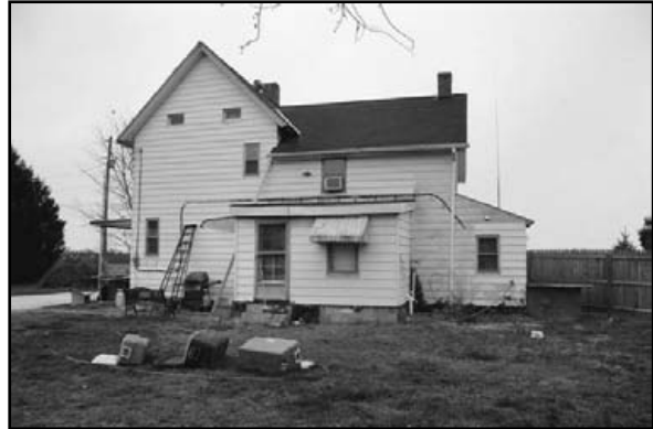
main building (.001) east side , view to W
