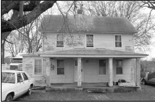
main building (.001) facade, view to S
