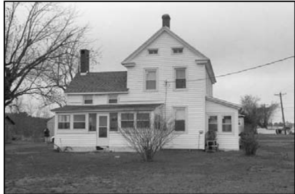
main building (.001) east side, view to W
