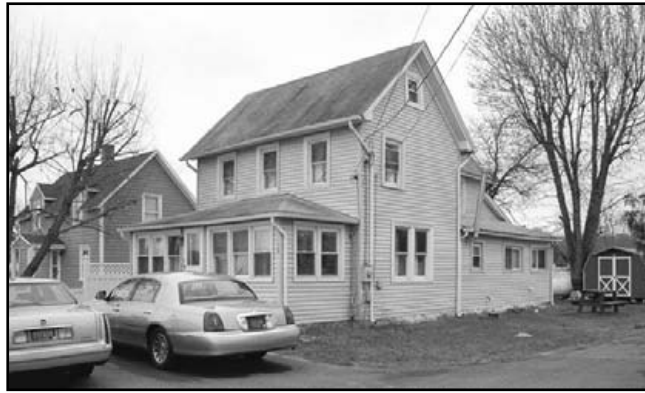
main building (.001) façade and west side, view to SE
