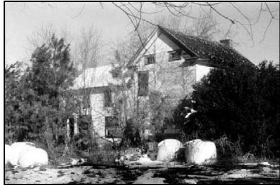
main building (.001) rear, view to NE
