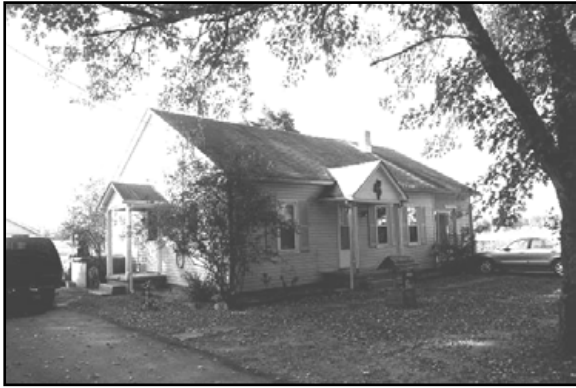
main building (.001) façade and east side, view to SW
