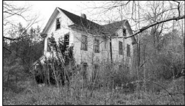
main building (.001) rear and north side, view to SW
