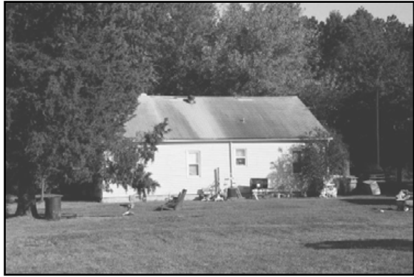
main building (.001) rear, view to NE
