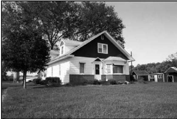
main building (.001) façade and south side, view to NW
