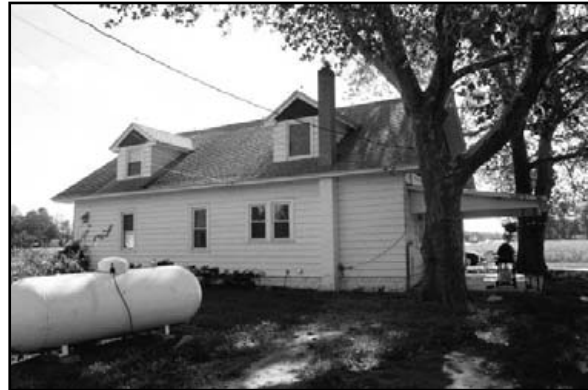
main building (.001) rear and north side, view to SE
