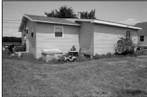
main building (.001) rear and west side, view to NE
