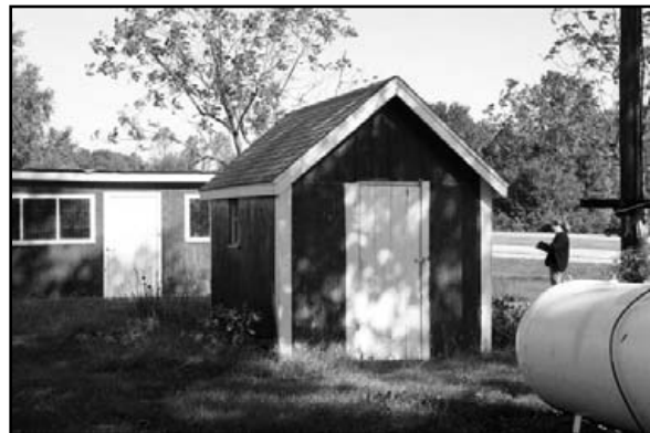
smokehouse (.003), view to NE
