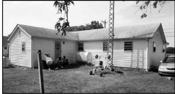
main building (.001) rear and east side, view to NW
