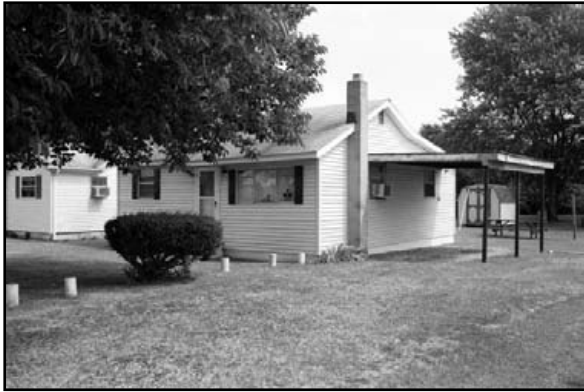
main building (.001) façade and west side, view to SE
