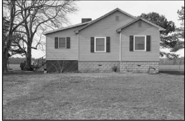
main building (.001) south side, view to N
