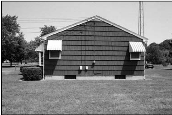
main building (.001) south side, view to N
