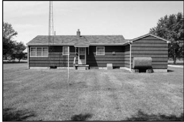
main building (.001) rear, view to W
