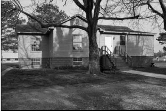
main building (.001) façade, view to E
