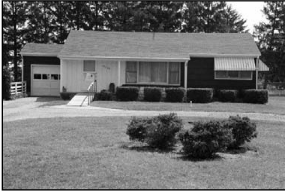
main building (.001) facade, view to E
