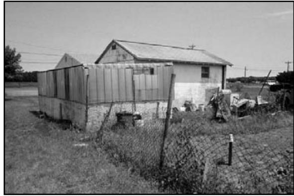
garage/storage shed (.002), view to NE
