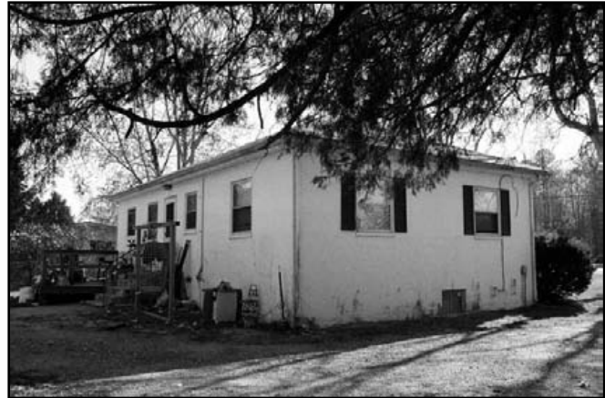
main building (.001) rear and north side, view to SW
