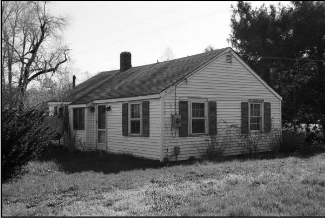
main building (.001) façade and south side, view to NE
