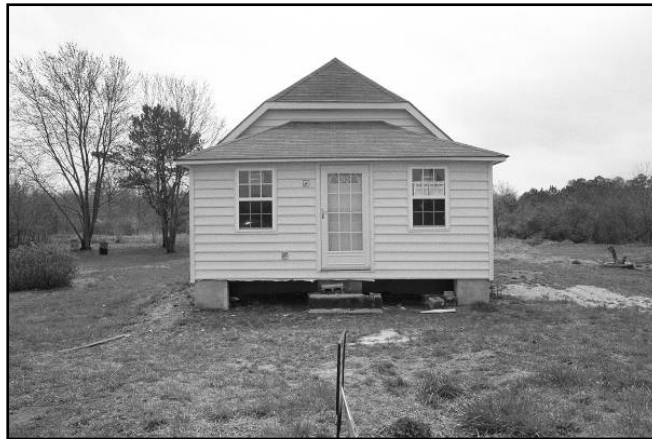
main building (.001) façade, view to S
