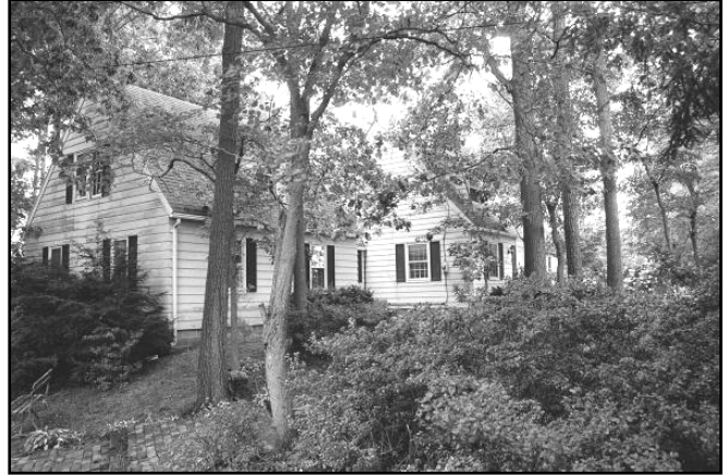
main building (.001), façade and north side, view to SE
