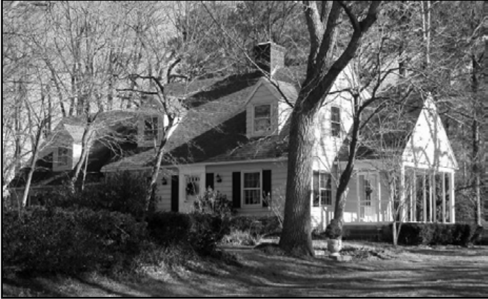
main building (.001), façade and south side, view to NE
