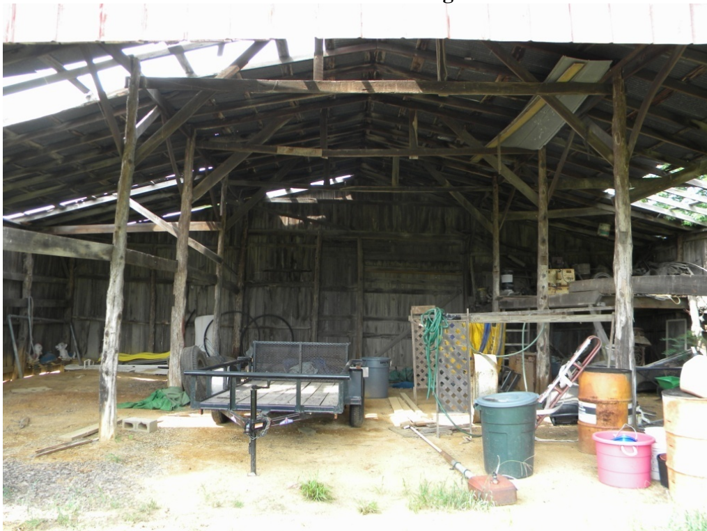
Interior detail looking north
