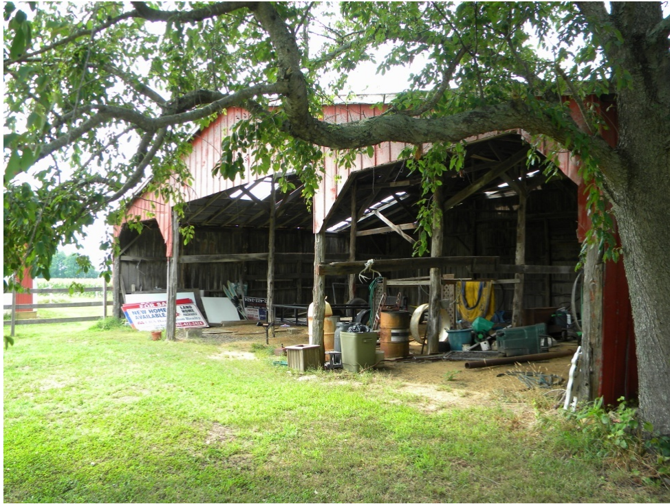
Three bay Machine Shed Storage Barn looking northwest
