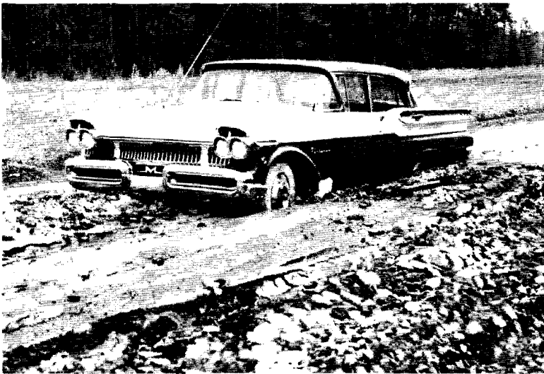
Road 224 in Sussex County, showing damage caused by prolonged cold weather.
