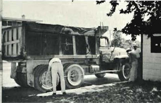
Checking truck weight and measurements helps control wear on highways.
