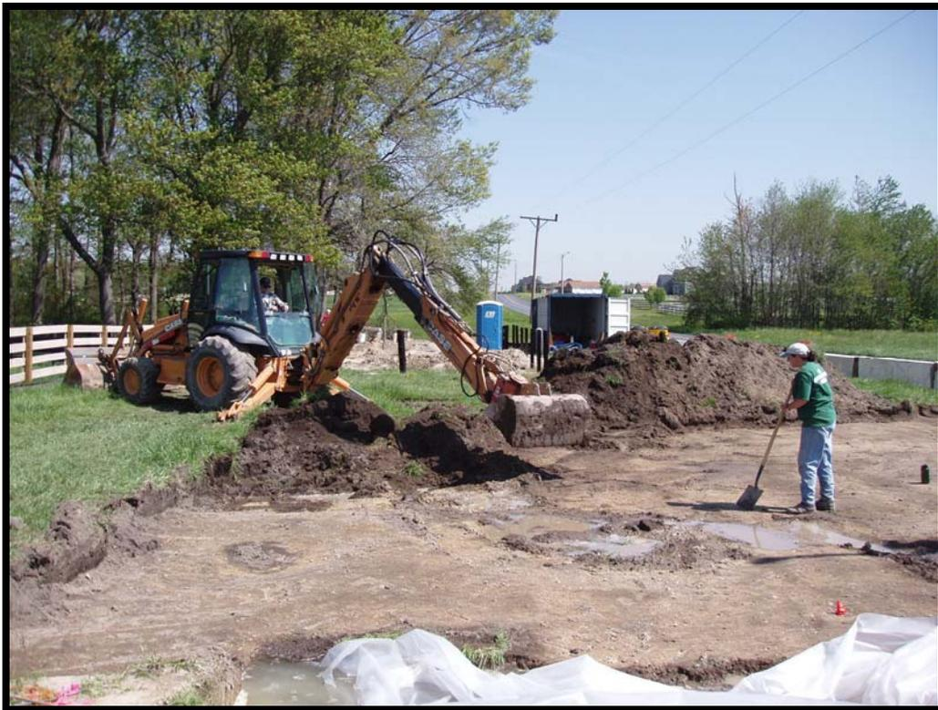
Figure 2.4 Backhoe stripping of the plowzone.
