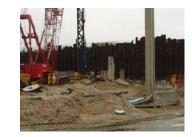
They start with driving individual concrete piles and then build a cap (footing) to cover each pile group. The pylon towers, which are the main vertical structures that hold up the bridge, are then built on top of the footing, and are where the bridge gets its stability and strength. The pylon towers cannot be constructed all at once, so engineers use climbing steel and wooden forms to work as they move up the pylon tower.
