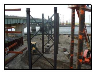
How do they build the center portion of the bridge over the Inlet? During construction of the center part of the bridge deck the bridge builder must construct what is called a *form traveler*. It is a movable form that will hold the rebar and fresh concrete to make the superstructure piece-by-piece.
