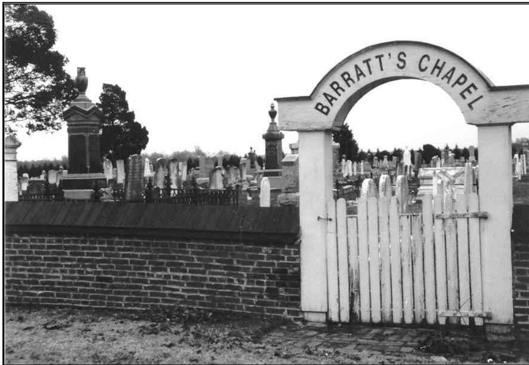
Barratt's Chapel cemetery gate, north elevation, facing southeast.
