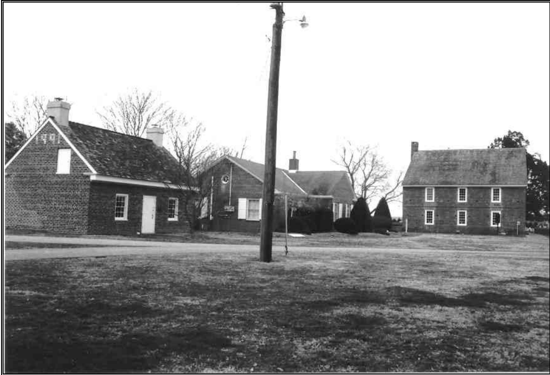
Vestry, museum, and Barratt's Chapel, north and west elevations, facing southeast.
