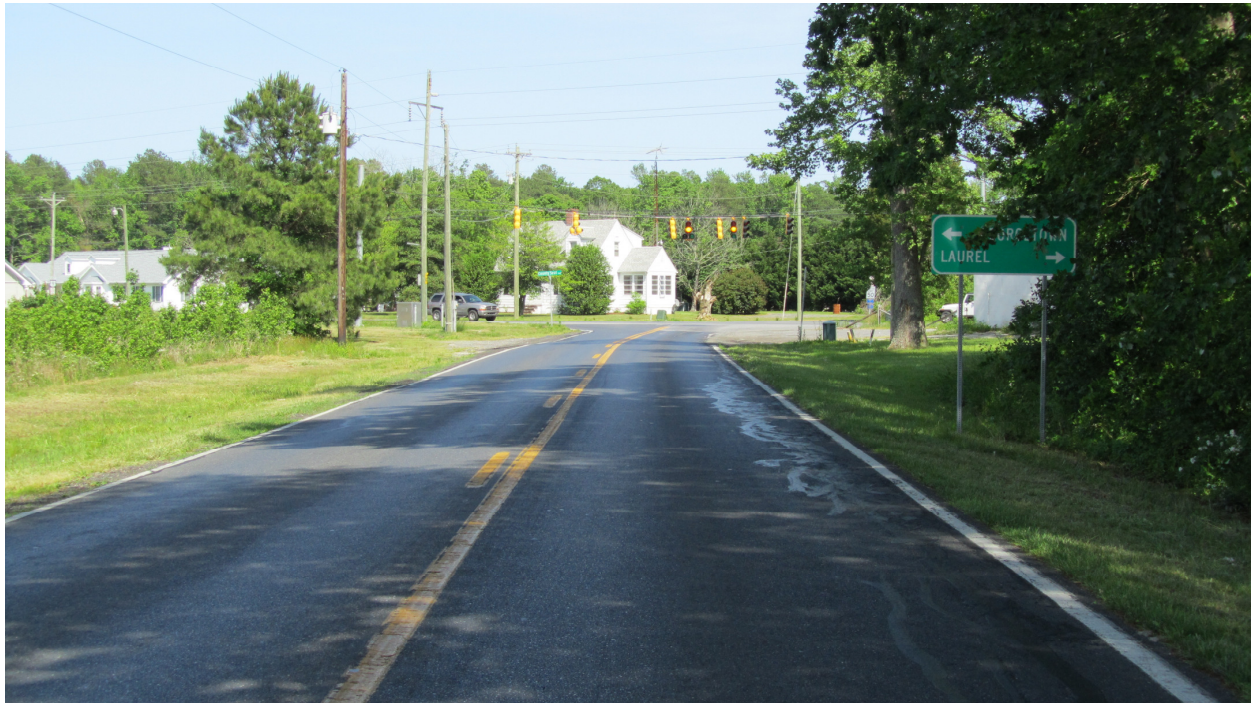
Photo 4: The Guide Sign Covered by Tree Branches on the Southbound Old Furnace Road Approach at US Route 9
