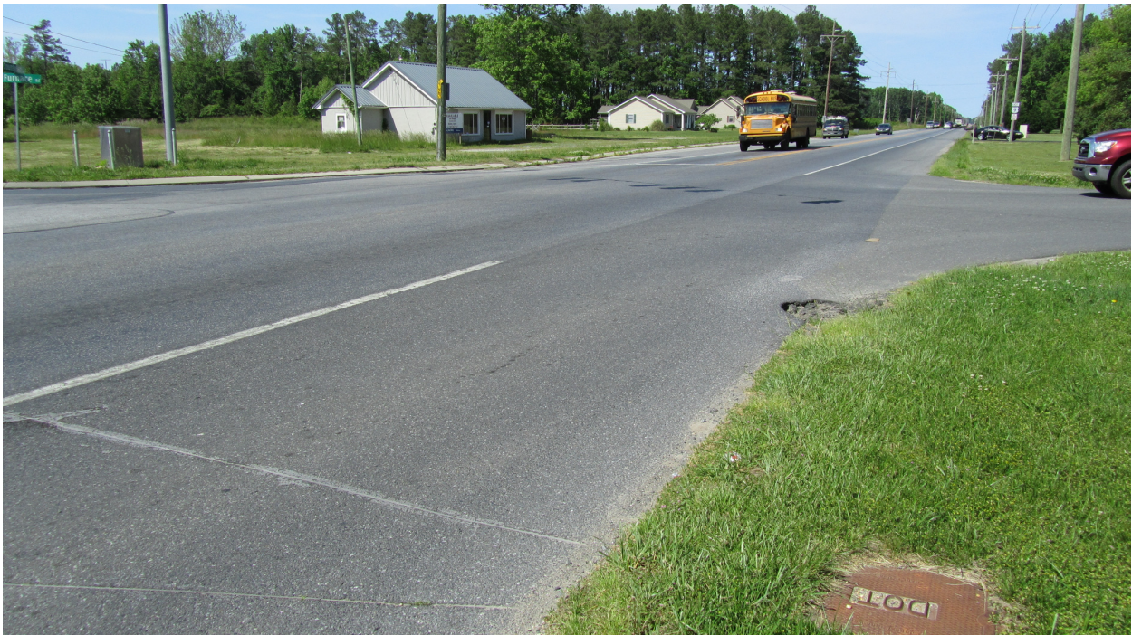
Photo 6b: A Pavement Breach on the Eastbound US Route 9 Approach at Old Furnace Road / Whaleys Corner Road (Looking East)
