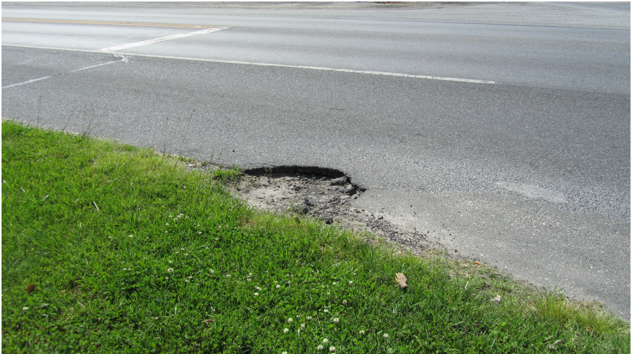
Photo 6a: A Pavement Breach on the Eastbound US Route 9 Approach at Old Furnace Road / Whaleys Corner Road (Looking North)
