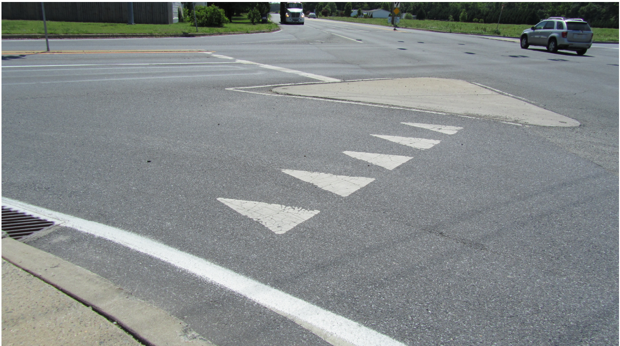
Photo 7: Existing Stop Bar and Shark Teeth Markings on Northbound DE Route 20 Approach at US Route 9 and DE Route 20 Intersection
