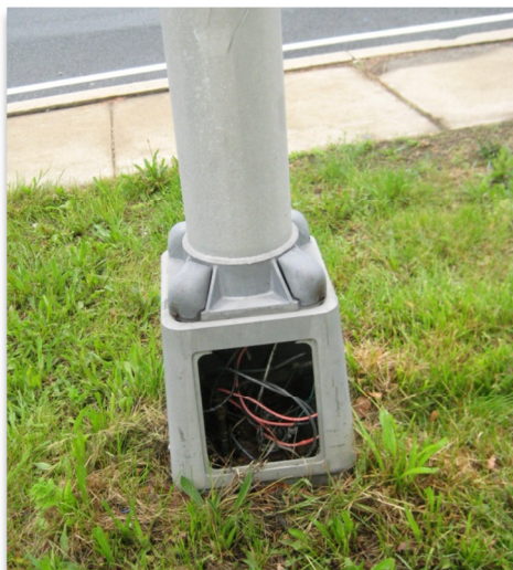
Photo 6: Pole #1702 Transformer Base Cover Missing
