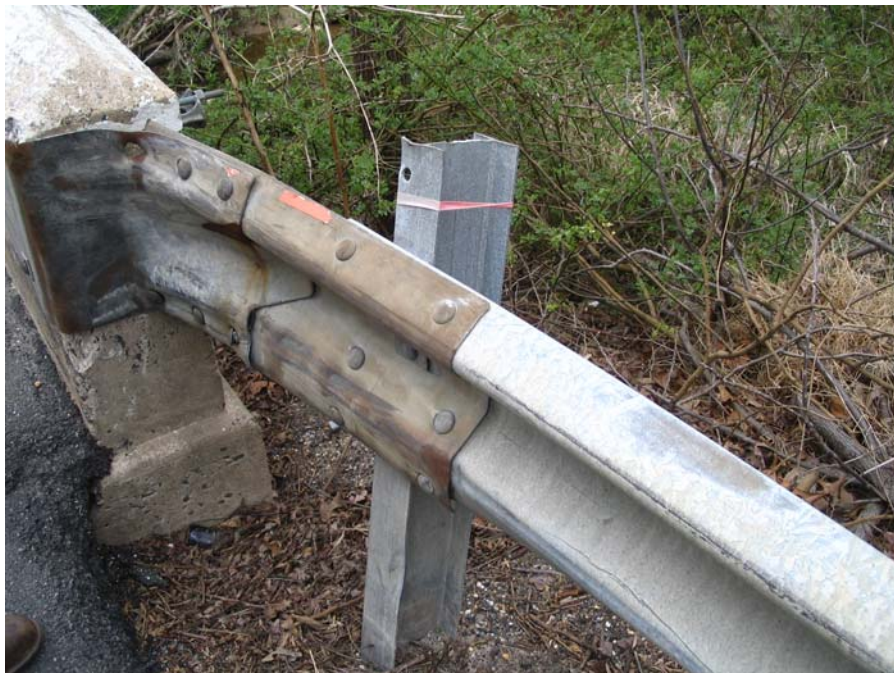
Photo 8: Damaged guardrail at leading edge of bridge parapet on the north side of Welsh Tract Road
