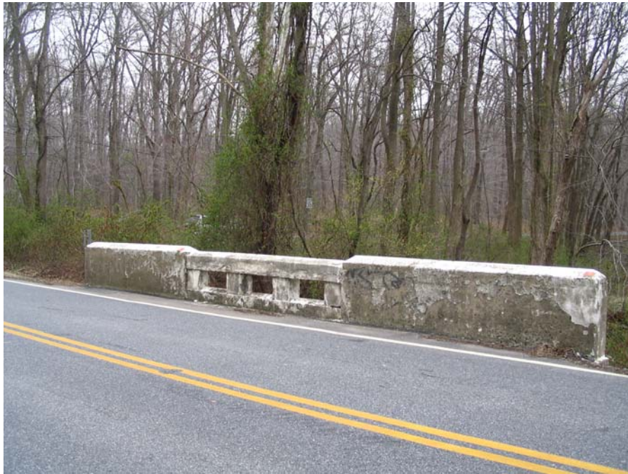
Photo 7: Welsh Tract Road at unprotected bridge parapet on the south side of the road
