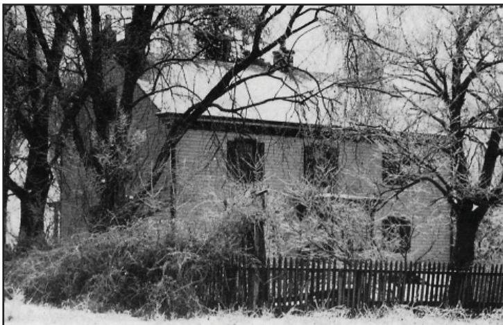
The back of the stone house as it looked around 1920. The stone has been covered with wooden siding.
