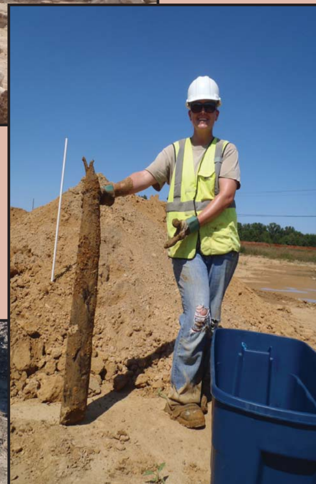
Representative pieces of the well cribbing were removed mechanically and by hand.
