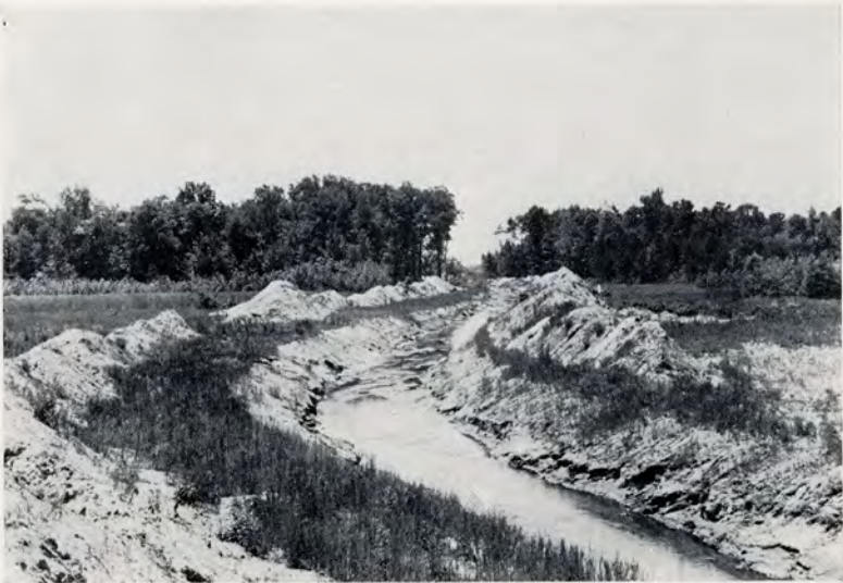
Figure 25—A drainage project in class III land.
