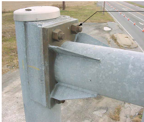
Bolted Connection
