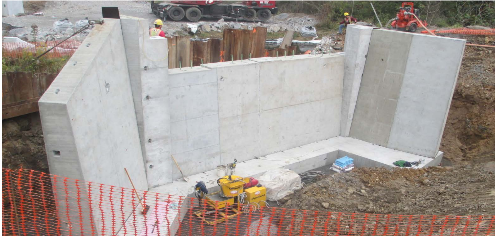
ABUTMENT – COMPLETED PRECAST ASSEMBLY
