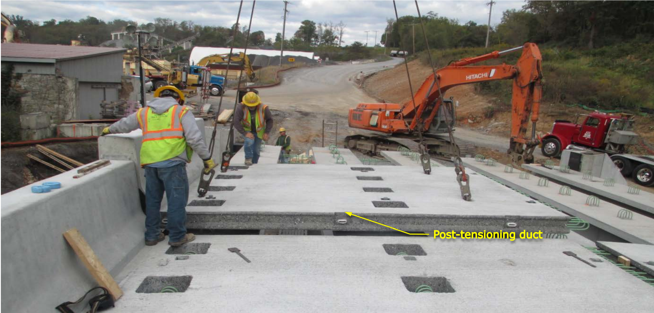
PRECAST DECK PANELS
