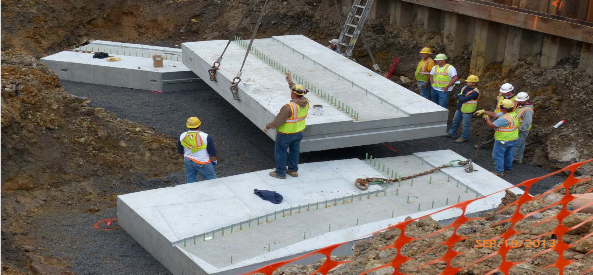
ABUTMENT – FOOTING INSTALLATION
