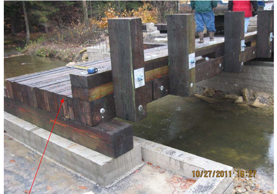
Timber Super Being placed
