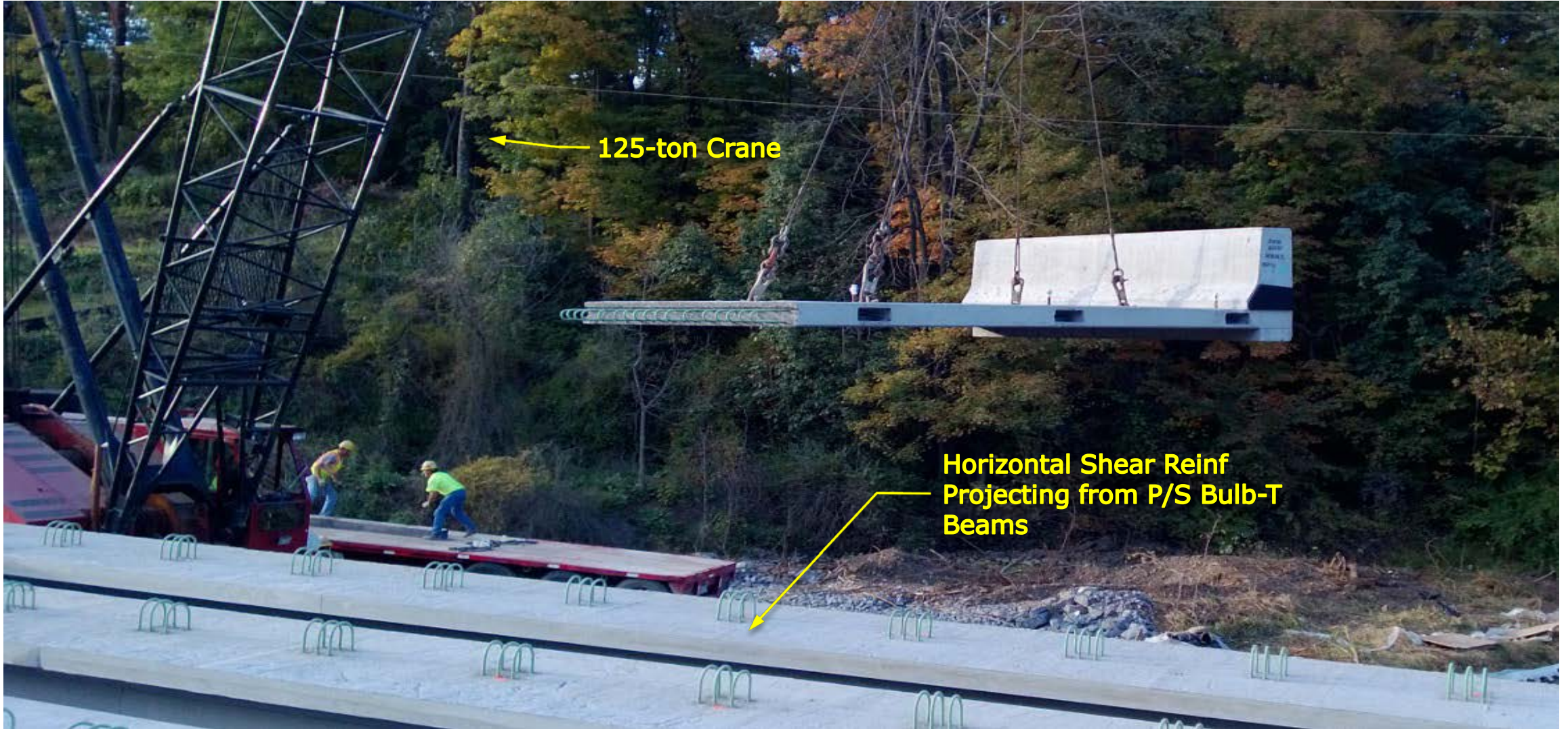
PRECAST DECK PANELS
