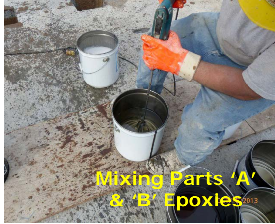
PRECAST DECK PANELS Epoxy Grout in Beam Haunches & Shear Pockets
